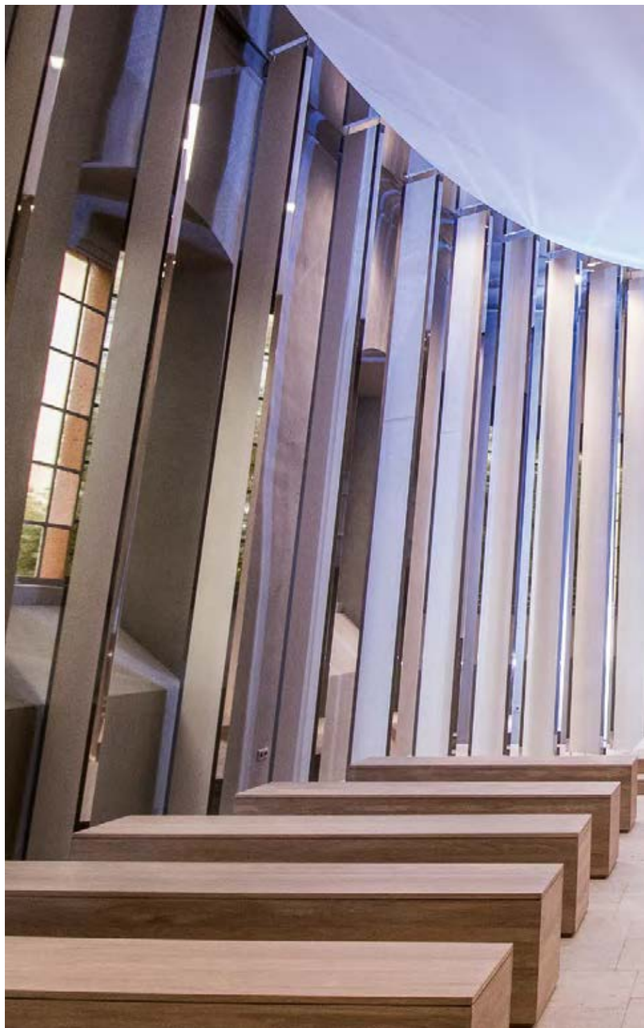
TECHLAM® Basic Ice Chapel in Castle Leuchtenburg Leuchtenburg, Germany
